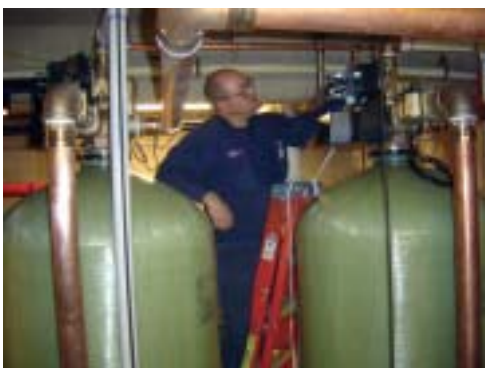
Andrew McDougall adjusts a newly installed unit.
